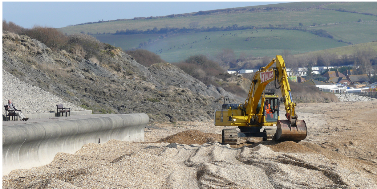
Beach replenishment at Overcombe Beach, Weymouth. Copyright: Dorset Coast Forum
